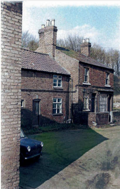
N.B. Drained Pinxton Canal just behind the hedge.
