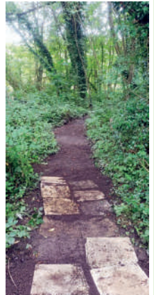
Path improvement work
