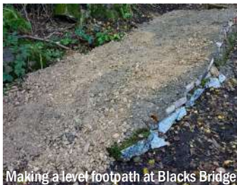
Making a level footpath at Blacks Bridge.
