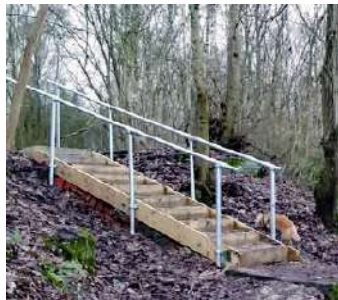
The new steps before the lower hand rail was fitted.
