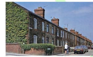
Forge Row built from iron slag stone (known locally as Rodneys), still lived in after over 200 years.
