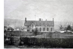
The Mechanics Institute, now known as Butterley Court, was designed by Henry Isaac Stephens in 1846 probably Derbyshire's most prolific and accomplished architect at the time.
