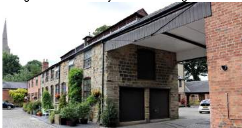
Park Mews is the new name for the residential conversion of farm buildings at the former Riddings Farm.
