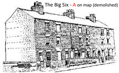
The Big Six - A on map (demolished)
