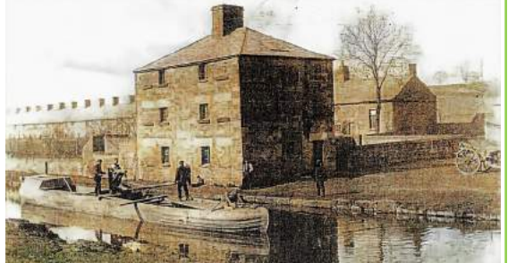
Photograph showing a barge on the canal in the late 1800's to early 1900's. Behind the large building in the front is No. 50 which is the last house in Stone Row.
